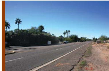
Existing Lincoln Drive
